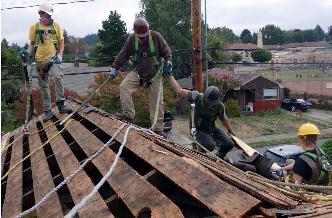
Deconstruction Crew, Portland, OR (Photo: City of Portland)
